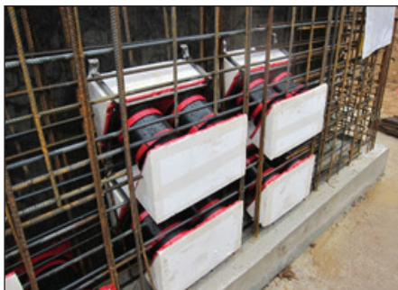
HSI 150-1x2 K2 S30°/300 (prije betoniranja)
