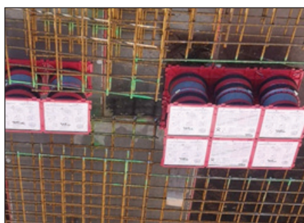
HSI 150-2x3 K2 Varia/260-365 (prije betoniranja)
