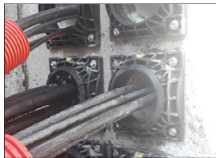
Brtvljenje NN kabela kroz HSI 150-DFK i HSI 150-DG-3/24-54
