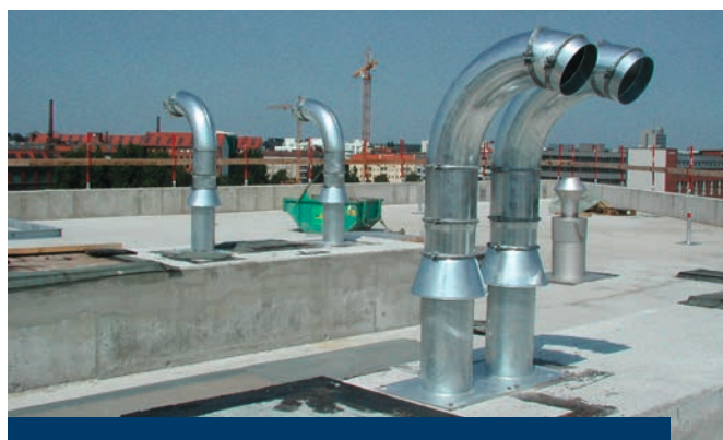
installed SHD 200 before installation of the flat roof seal
