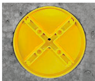
Protective cover after grouting in concrete
